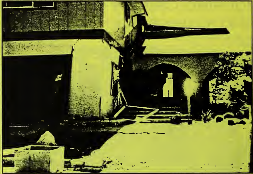
This single family home, very similar to many houses in the Bay Area, saw extensive damage in Southern California. (Courtesy of Degenkolb Associates.)
